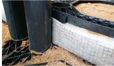
Use the TPGeoGrid to bridge the height in subbase material.
