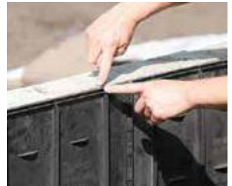
The top of the panels should be above the soil surface around the tree.
