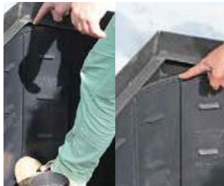
In a open tree pit, the panels should be placed as close as possible to the kerbing. This way you create the maximum space for the tree
