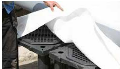
If the height difference is less than 20 cm you can use the standard TP geotextile on top of the system.
